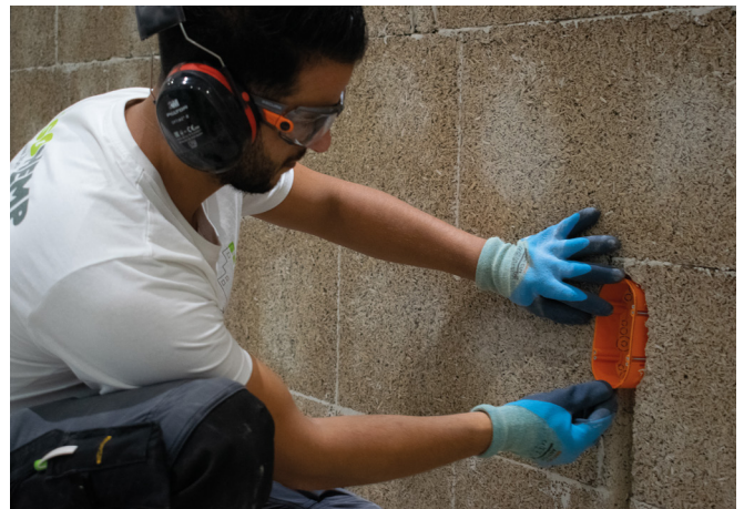
4 Collect the waste from your hemp block cuttings and grind it. Then mix it with ProKalk binder at a 50/50 ratio. Moisten the resulting mixture with water to obtain a homogeneous, slightly moist mixture. Fill the cavities with the mixture.
