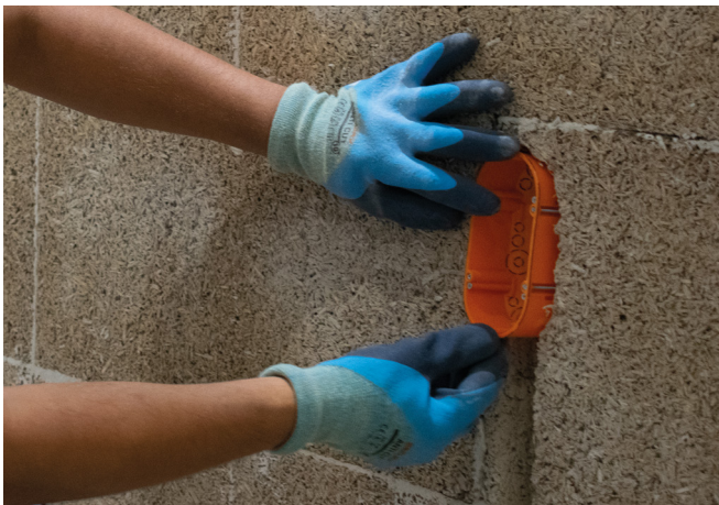
3 Fix the boxes and electrical cable ducts.
