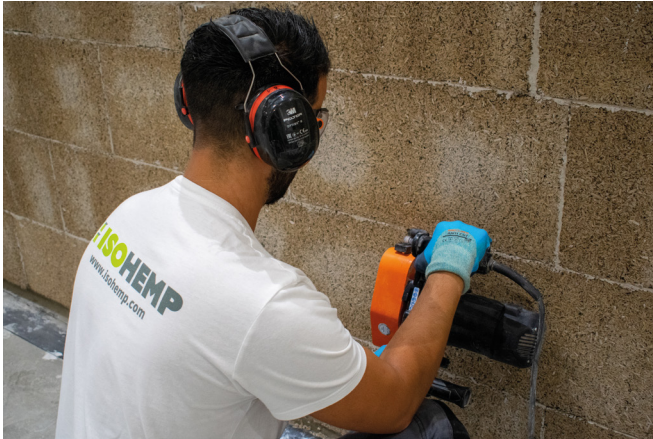
1 Create the grooves using a grooving machine.
