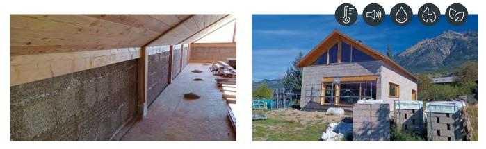
**Project:** To move away from the stereotype of the mountain chalet with wooden framework and vapour barrier, the architect recommended IsoHemp blocks to the client. This material was the perfect answer to the project's requirements: distributed thermal insulation, easy to install, retaining its breathable properties and easy application of plaster on both sides, also allowing partial self-construction.
