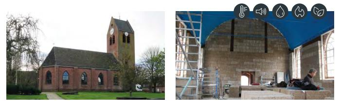
Project: Renovation project of a former church to bring it up to low-energy standards. Interior insulation using hemp blocks (30 cm thickness). Wall heating and interior finishing with clay.
