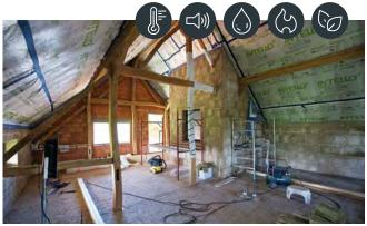
Project: Renovation of an old farmhouse with a timber framework filled with hemp blocks. Along the inside, the farm was walled up with hemp blocks of 15cm thickness. This solution prevents condensation problems and damage to the wooden roof truss.
