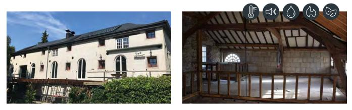
**Project:** Complete interior renovation of an old barn using 15 cm thick hemp blocks. The aesthetic character both on the inside and on the outside of the former farmstead is preserved, and potential condensation problems are avoided, thus leaving the wooden roof unaffected. Along the inside finished with natural plaster based on lime.
