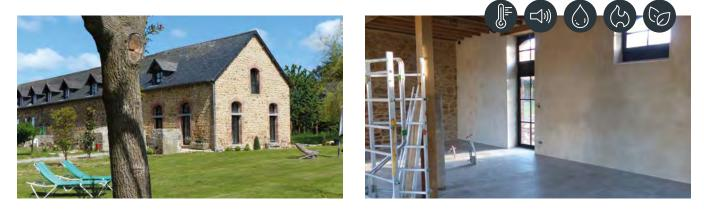
Project: Renovation and restoration of the inside of a former French 'longère' (longhouse farm, which in this case served as a pig farm) using 20cm hemp blocks. Preserving the external character of the building with old authentic stones. Plastered on the inside with lime.
