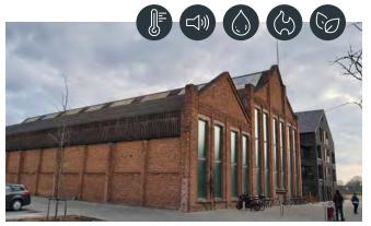
Project: Construction of 8 storage rooms for the preservation of works of art of the city of Mechelen. This project has a "box in a box" structure with walls of 30cm thick blocks and between 6m and 8m high. A total of 1500m<sup>2</sup> of hemp blocks were used.
