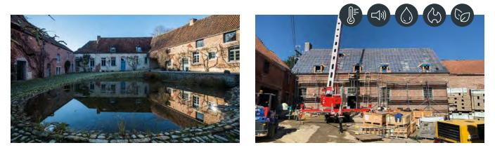
**Project:** Conversion of a heritage farmhouse into a hotel. Insulation was carried out from the inside to preserve the façade. The hemp block provides efficient moisture control to avoid problems such as cold bridges, condensation points, dew points, ... It also guarantees the preservation of the old, classified building.
