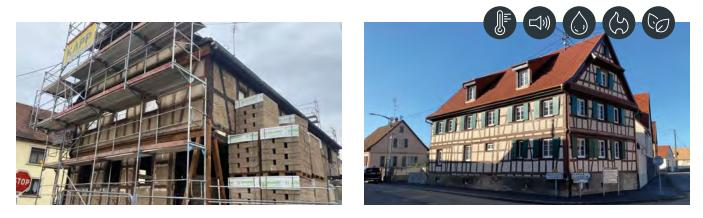
**Project:** The heritage of the Alsace region is of great historical value and must be preserved. The renovation of a half-timbered house is a technical challenge where many parameters must be taken into account, including thermal insulation and moisture regulation so as not to damage the wooden framework. In this case, hemp block are the obvious solution, as it stays close to the know-how of the past.
