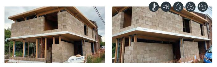
Project: Construction of a single-family house in wooden post-and-beam system with hemp blocks for this zero-carbon project. The clients wanted high energy performance and a future-ready house. They chose hemp insulation with hemp blocks of 42cm thickness
