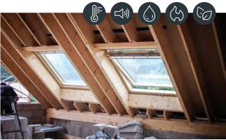
Project: New construction of two very low energy houses with a structure of wooden posts and beams that was completely walled with only 42 cm thick hemp blocks (12 cm + 30 cm). Exterior finish based on lime.
