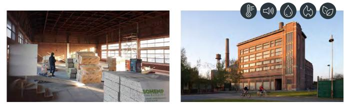
Project: Renovation of nearly 1,000m<sup>2</sup> of a classified former power station into a coworking and event space. The insulating shell was made with 15cm hemp blocks to provide acoustic and thermal comfort while respecting the heritage.
