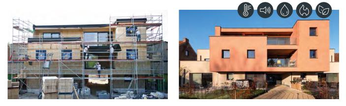
Project: A new apartment building built with CLT and an outer shell of 30 cm thick hemp blocks. The client was looking for natural and breathable insulation. The interior walls consist entirely of 12 cm thick hemp blocks that significantly improve the acoustics of the living spaces.
