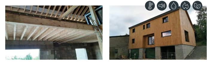
Project: The Hempro system proved to be the ideal solution for the building envelope in this project to meet the specific low energy requirements of the building. It is used in combination with a system of concrete beams and columns.
