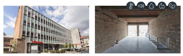
**Project:** For the interior renovation of a former two-story office building, 15 and 30 cm hemp blocks were used to transform the building into 9 lofts that meet very low energy standards. The entire inner shell was made of hemp blocks which were also used for the double partition walls. Result: optimal sound insulation and fire-resistant walls. The natural interior plaster of IsoHemp was also used as a filler layer for interior walls.
